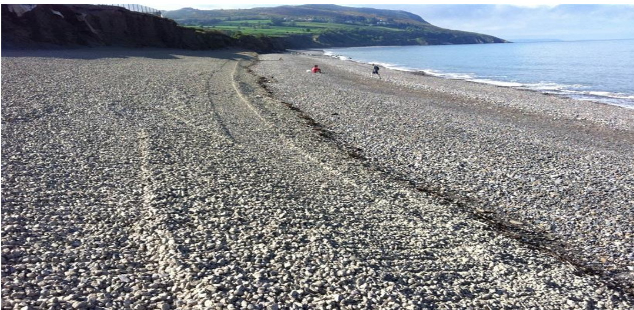
Completed beach nourishment works at Greystones North Beach. Site visit 25 May 2014
